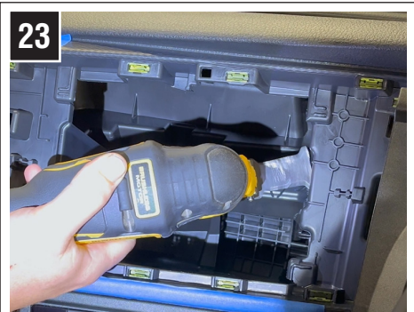
23 Use a multitool or reciprocating saw to cut the panel. Once removed, discard the panel, as this will not be needed again. Ensure the area that is being cut is clear of any wires.
